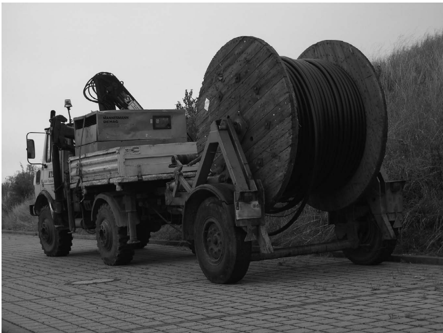
FIGURE 7.11 A cable drum in roadwork
